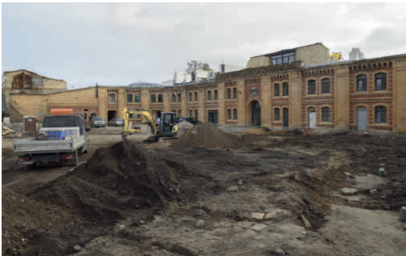
Construction work in the courtyard of *Kavalier Scharnhorst*; the layer of earth covering the roof has been removed
